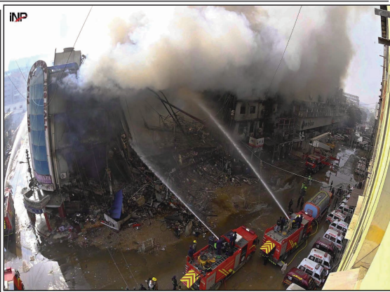
KARACHI: Rescue officials try to extinguish a fire at Gul Plaza. Authorities have confirmed six deaths so far, including a firefighter, after the fire erupted on Saturday night at the mall located a MA Jinnah road.
